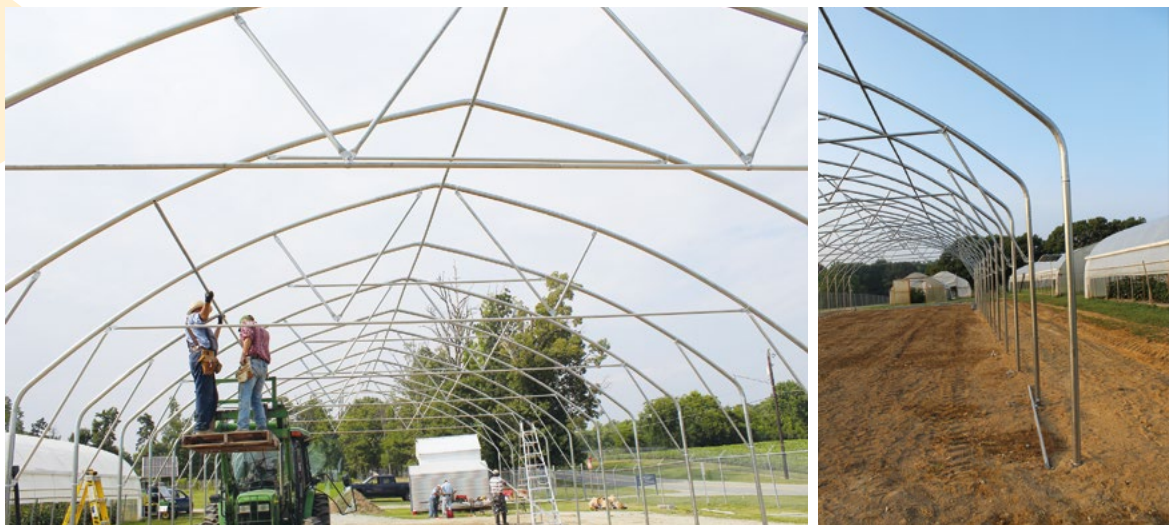
Picture 2-6: Connecting bows with purlins and installing w-trusses and braces.
