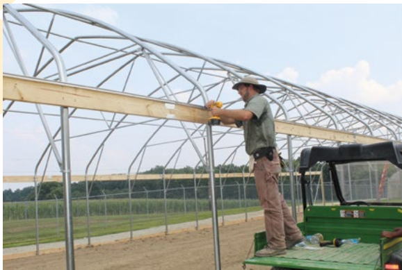
Picture 2-8: Installing c-channels on the hip board.
