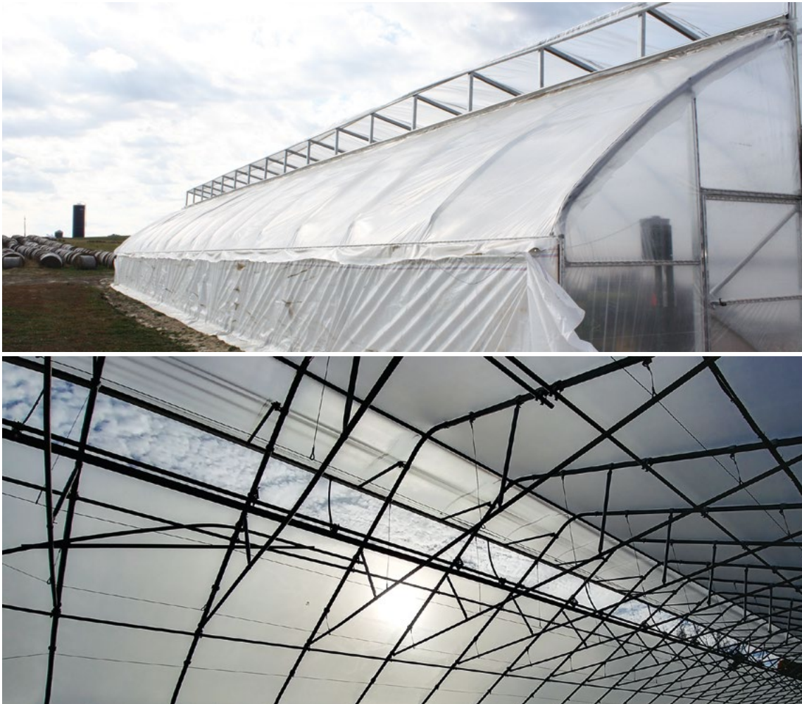
Picture 8-2: High tunnels with ridge vents. Top shows the Zimmerman brand and bottom shows a ridge vent by the Rimol Greenhouse Systems.
