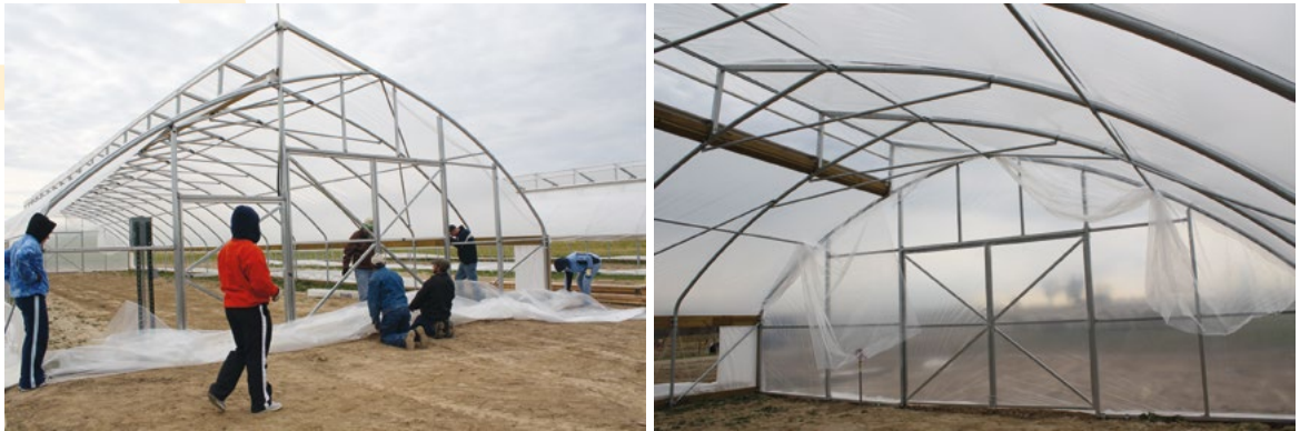
Picture 2-18: Putting plastic on end walls from the bottom (left). Plastic is secured into c-channels on the end wall with wiggle wires. The photo on the right shows a completed end wall before cutting the extra plastic.
