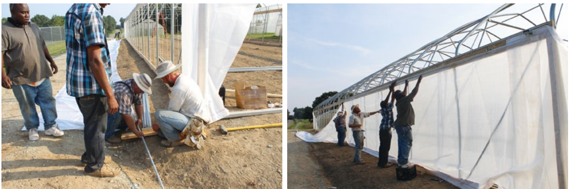
Picture 2-10: Attaching corner curtains (the white curtain in the left photo), inserting metal rod into the curtain (connecting rods as a rod is about to be inserted into the curtain), and attaching the rod with strings to the hip board through pulleys.
