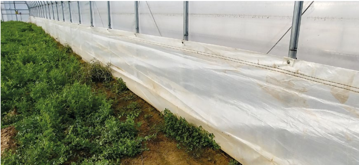
Picture 8-6: An extra layer of side wall fabric adds insulation to a high tunnel in winter.
