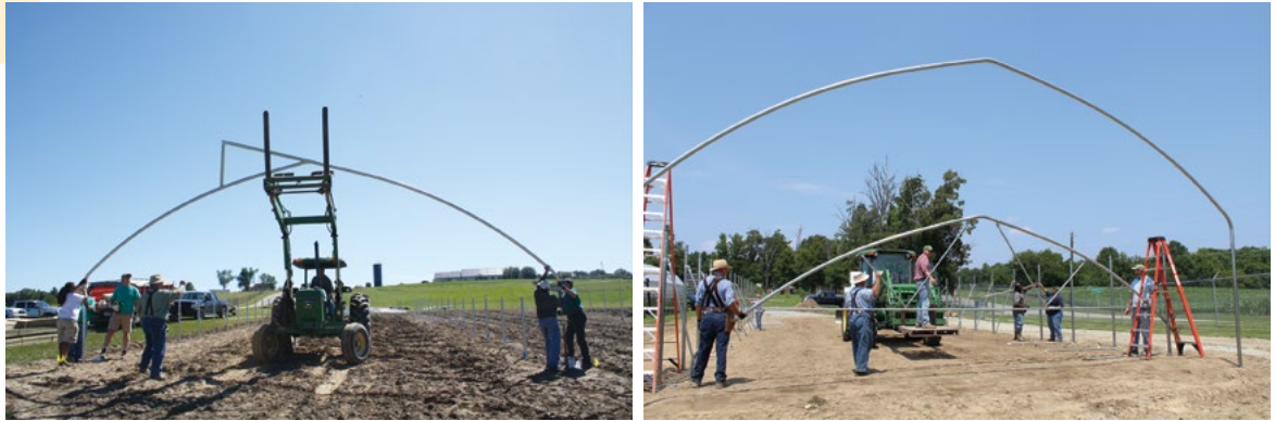
Picture 2-5: Connecting bows onto the side posts.
