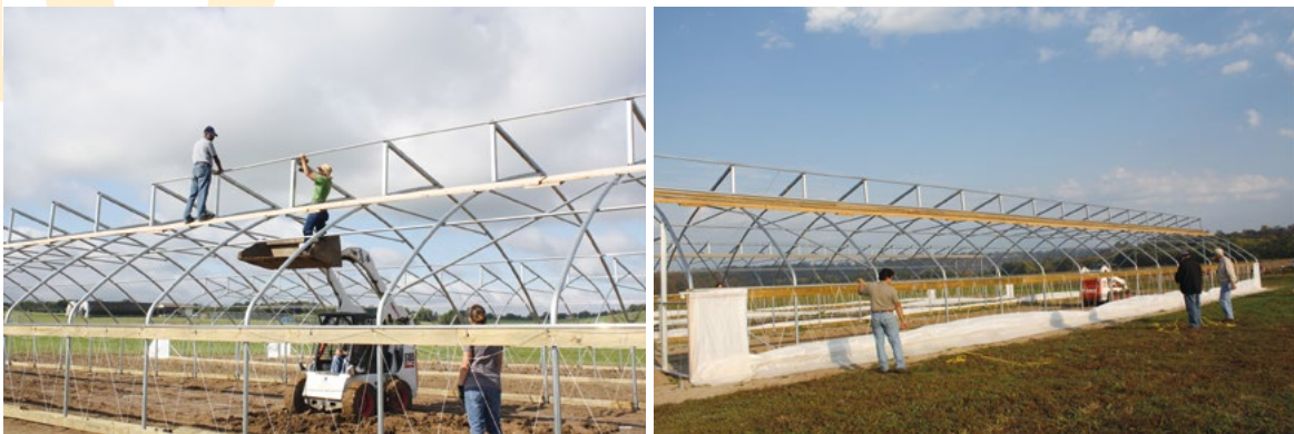
Picture 2-12: Installing ridge vent.
