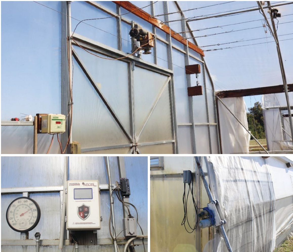
Figure 8-3: Temperature controlled automatic ventilation systems used on high tunnels at the N.C. A&T University Farm. In the top photo, one motor controls both curtains; in the bottom photos, each curtain is controlled by one motor.
