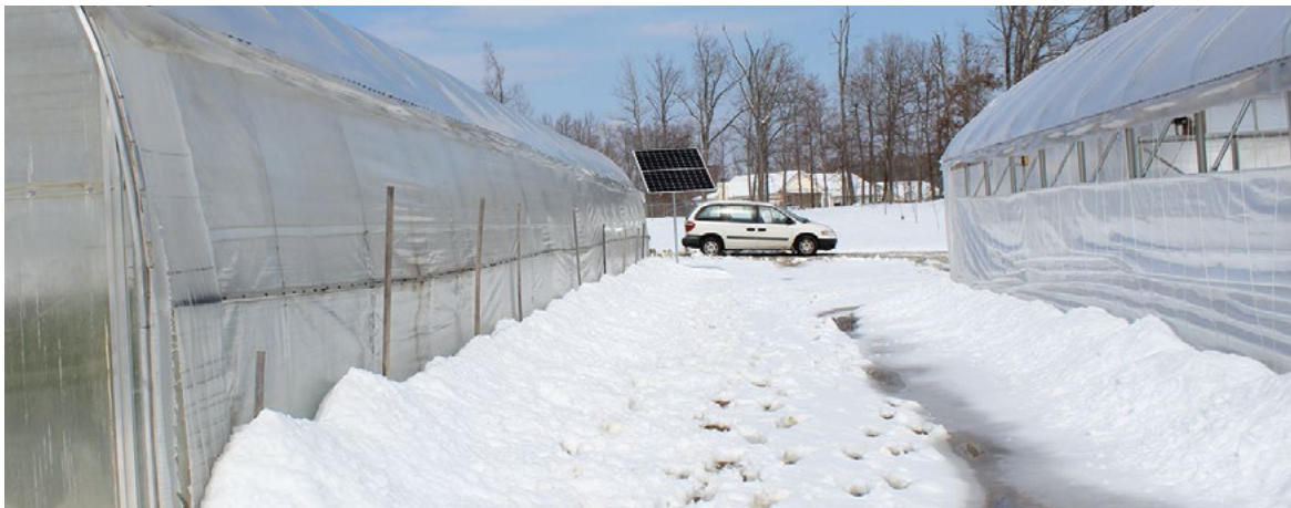
Picture 8-12: Snow piled up along the side walls prevents ventilation with a roll-up curtain (left), but not with a drop-down curtain (right).
