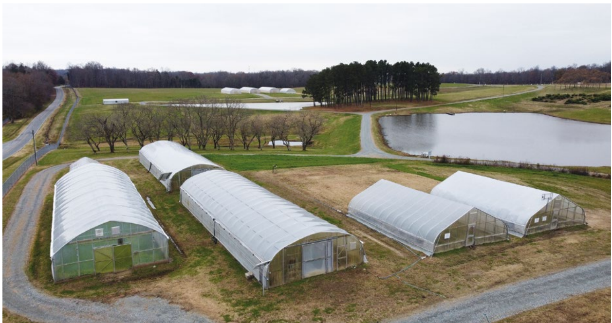
Picture 1-3. Single-bay high tunnels at the N.C. A&T University Farm. From left to right: A Quonset and gothic hybrid fixed high tunnel, two Quonset fixed high tunnels (tandem), and two gothic moveable high tunnels (side-by-side). Photo by John Kimes.
