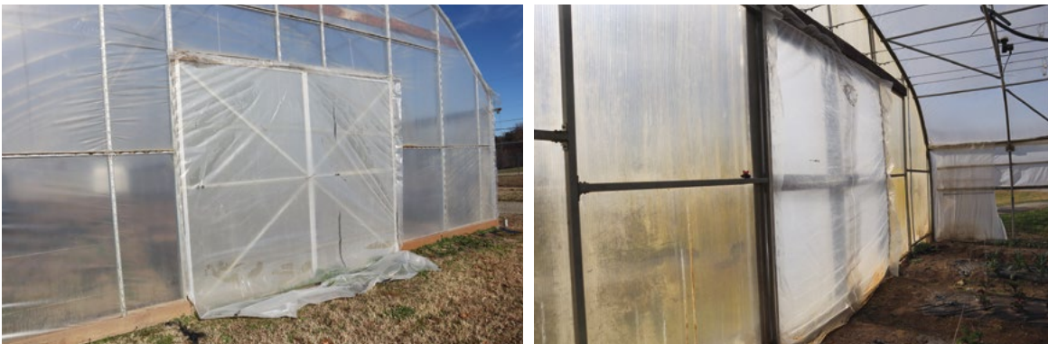
Picture 8-7: Extra plastic added to the end wall seals the gaps that leak warm air.
