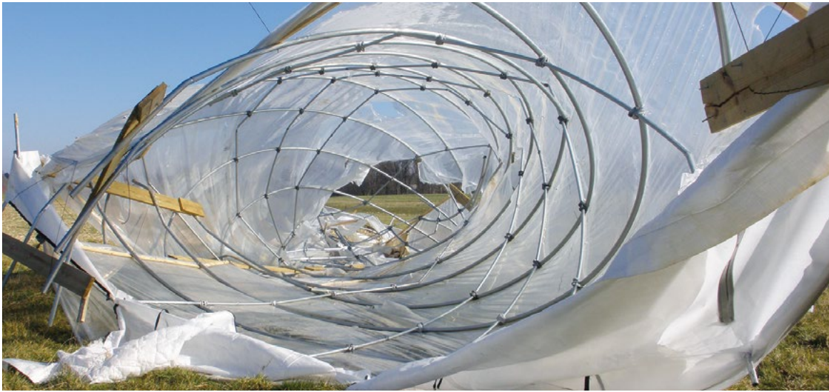
Picture 8-11: A high tunnel destroyed by a powerful windstorm. Photo credit: Dr. Tim Coolong.
