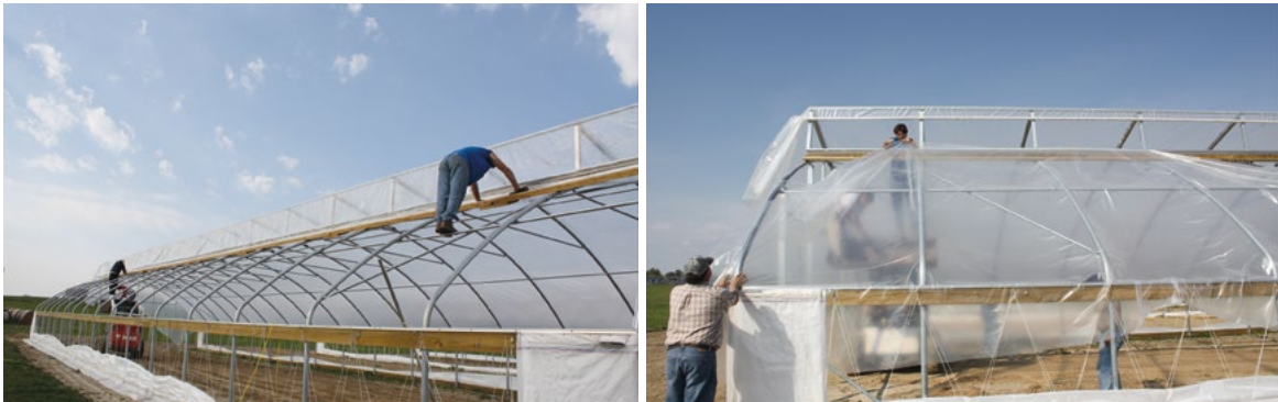
Picture 2-16: Securing the plastic film to the ridge vent (left), and putting on the second piece of plastic film.
