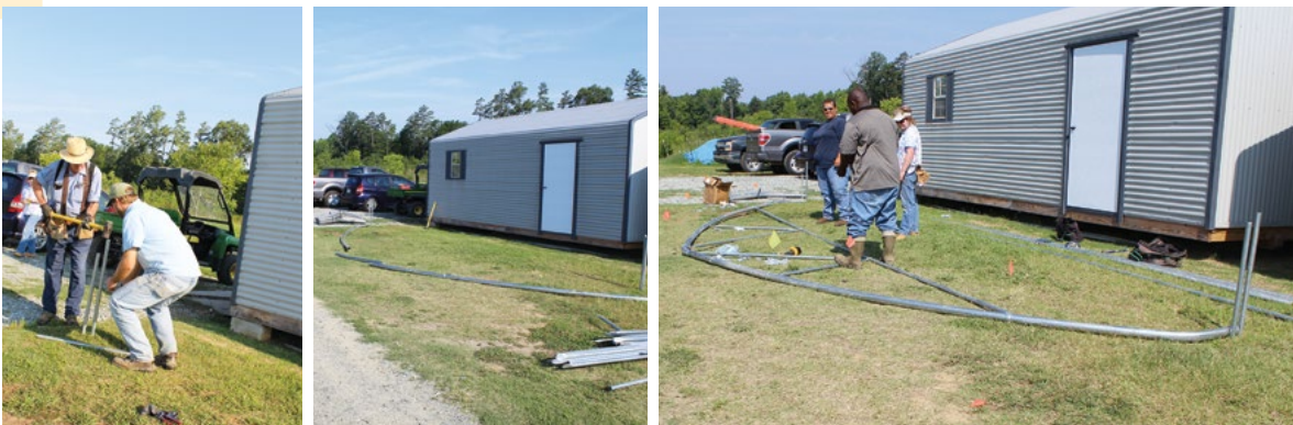
Picture 2-4: Assembling bows for high tunnel construction.
