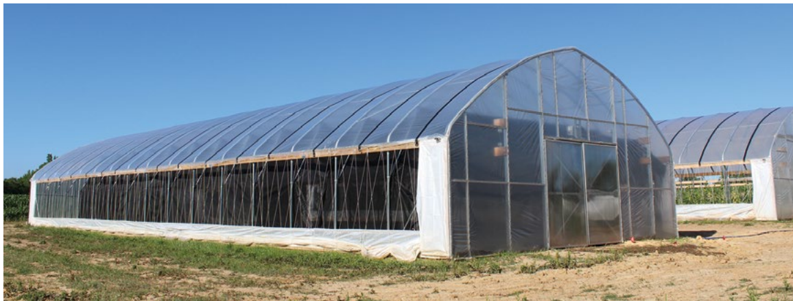
Picture 8-10: Straps installed over a high tunnel to hold the plastic cover tight.
